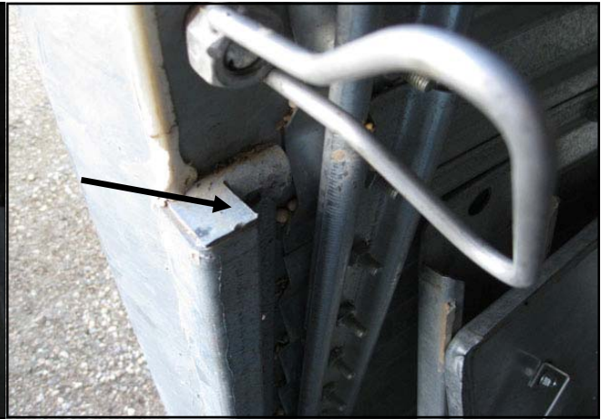
Metal Tab Cut And Bent Down
