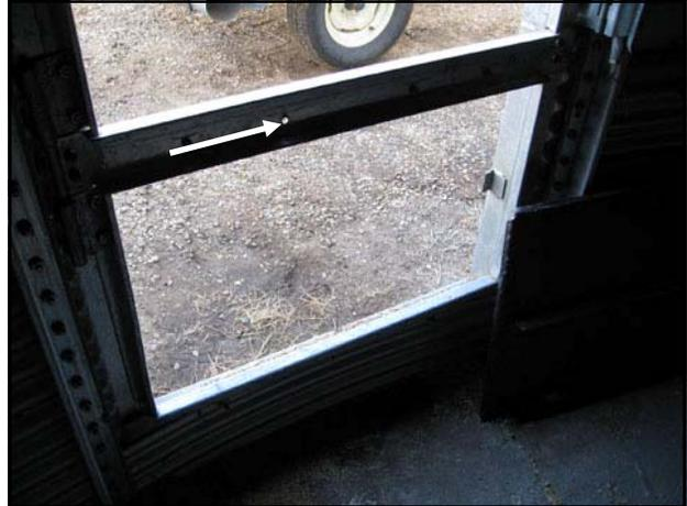
Open bolt hole in center bar
