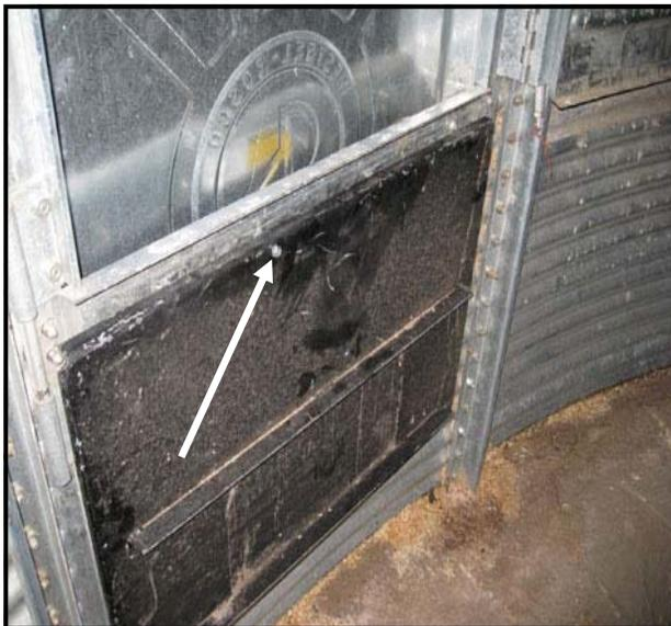
Attach with 3/8 x 2" bolt and nut enclosed
